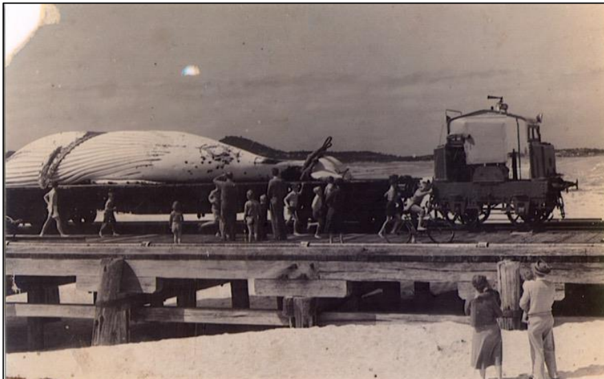
Figure 24: The whales were hauled from the jetty to the plant by rail. Shown here being pulled by the engine locally known as the green frog.
