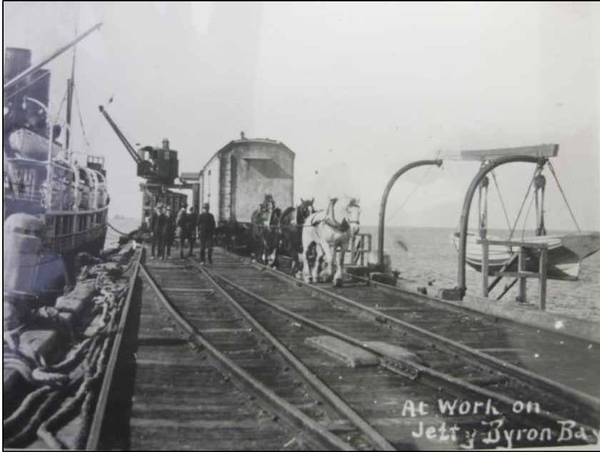
Figure 15: Undated image of the old Byron Bay Jetty. This is believed to be the original jetty which had been constructed prior to the establishment of the Tweed Railway and used a narrow gauge tramway. This photo appears to a date from the time after the conversion to standard gauge. ARHSnsw.
