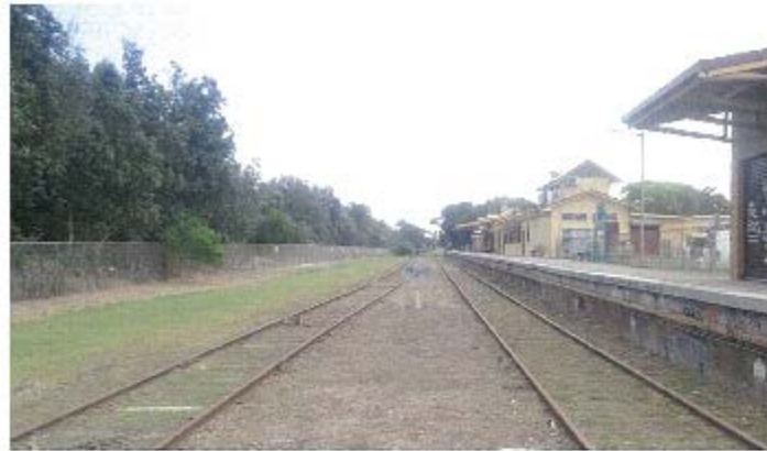
EXISTING VIEW looking east along the existing rail corridor and existing platform
