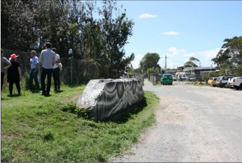
Figure 58: remnants of the concrete structure to the southern boundary and view to the pedestrian walkway.
