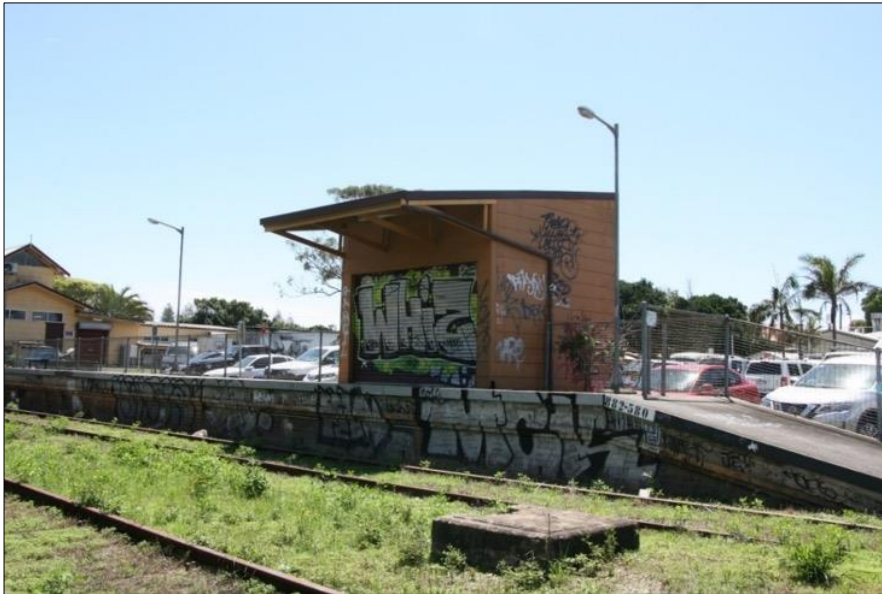
Figure 103 The western elevation of the Out of Shed Weir Phillips
