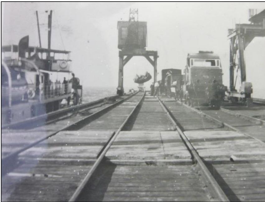
Figure 16: Undated image of what appears to be the second jetty which was designed for use with a standard gauge siding off the Tweed Railway. Note also the gantry cranes for loading and unloading boats. ARHSnsw.
