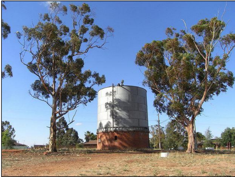
Figure 119: Brick and steel circular water tank Narrandera (Source Photograph by David Windeyer)
