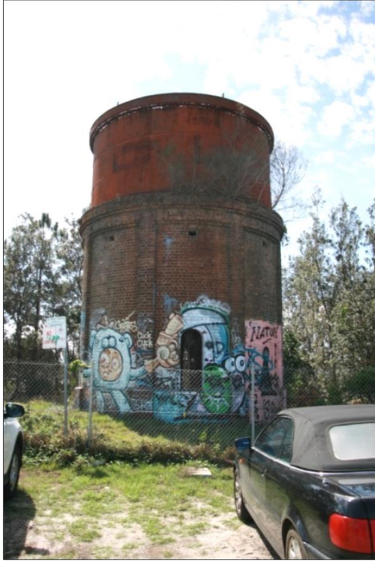
Figure 96 The water Tower as viewed from the west. Weir Phillips
