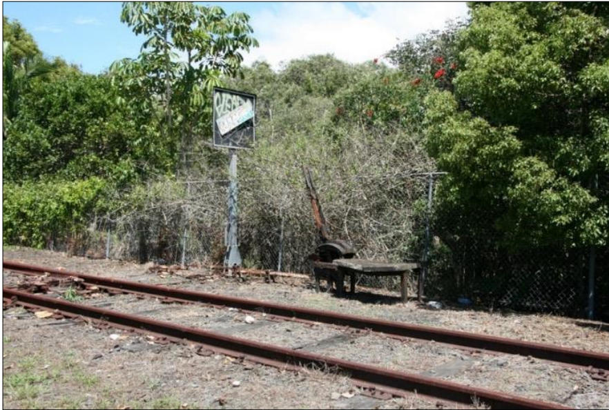
Figure 109: One of two surviving railway stitch levers. Weir Phillips
