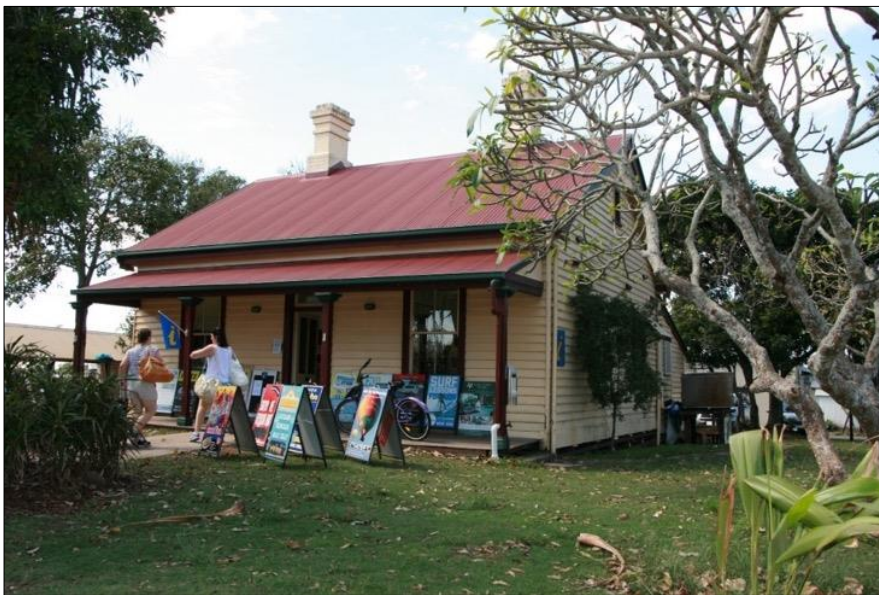
Figure 77: Northern elevation. Weir Phillips
