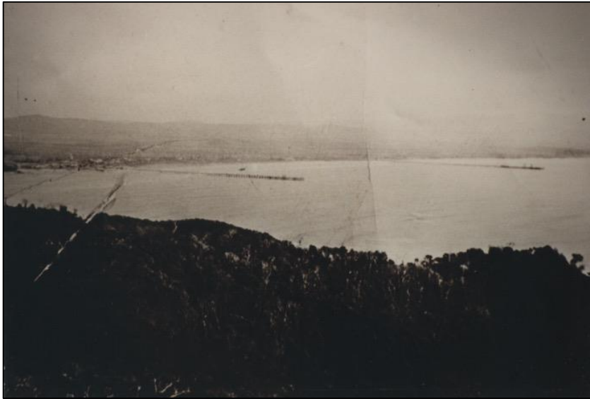
Figure 14: A rare photograph depicting both the old and new jetty.
