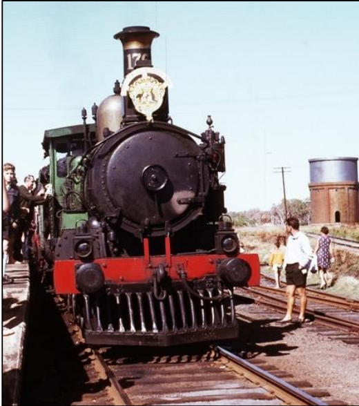
Figure 50: undated image of a steam train at Byron Bay with the water tower in the background. Note the siding providing access for the steam trains to the Water Tower.
