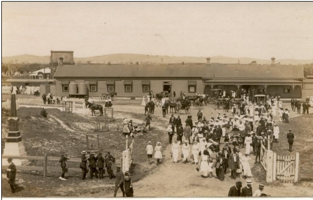
Figure 39: Victory Day March 1918 showing the station building, extended refreshment room and water tower. The war memorial remains has been relocated to the front yard of the Former Station Master's House. The gate posts, gate and fence to the eastern boundary have been removed. Photo courtesy of EJ Wright Collection, Byron Bay Library
