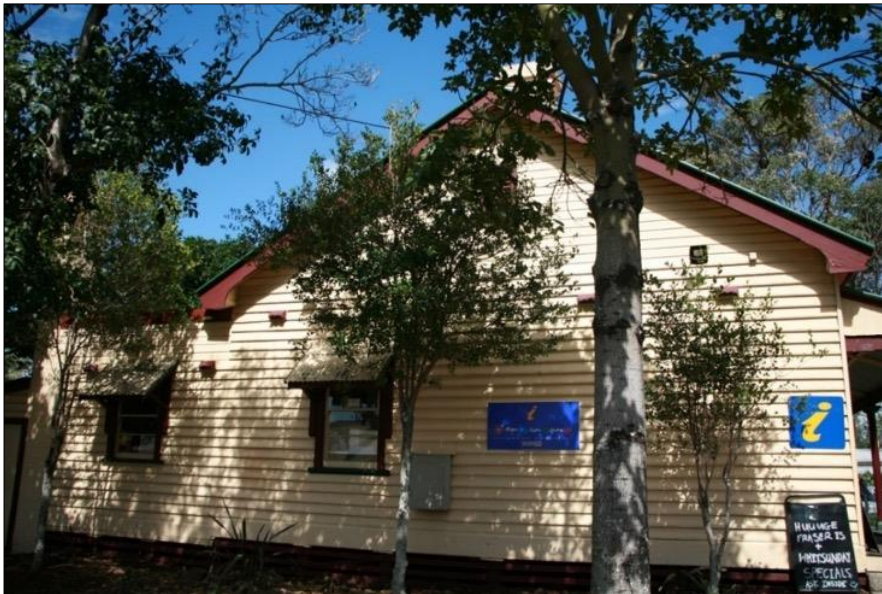
Figure 79: Eastern Elevation showing the simple timber barge detail. Weir Phillips
