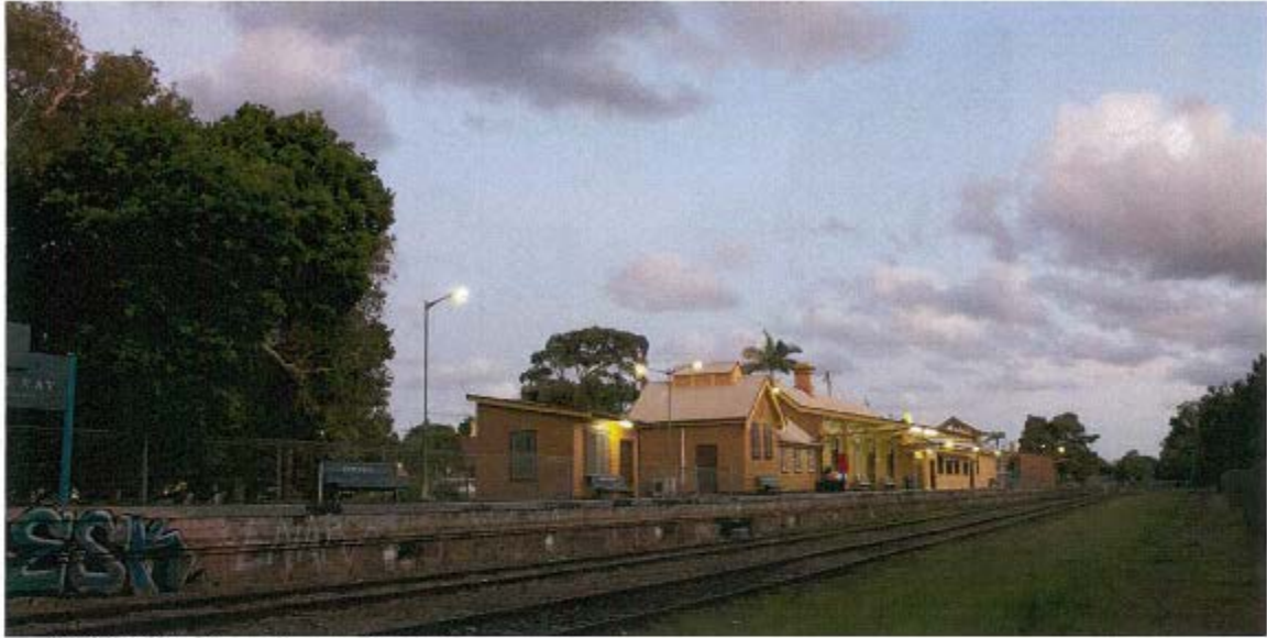
EXISTING VIEW: looking south past the railway station
