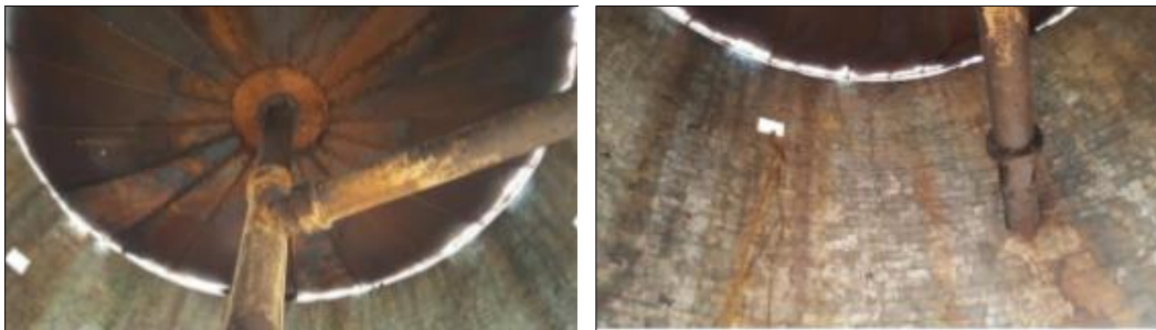
Figure 99 and Figure 100: Interior of the Water Tower. GHD Pty Ltd
