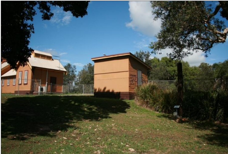
Figure 102: Rear of the Signal Box Weir Phillips
