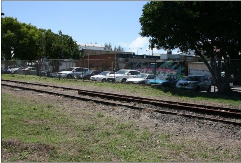
Figure 62: View to Lawson Street South Car Park to the north east corner of the site Weir Phillips
