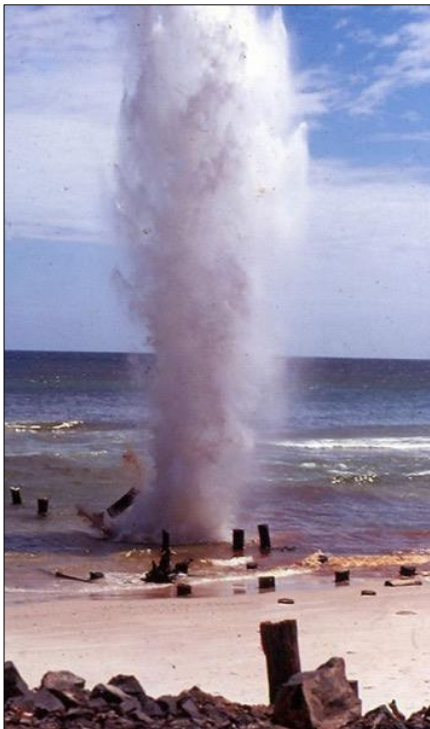
Figure 18: Demolition of the jetty. Max Prendergast.
