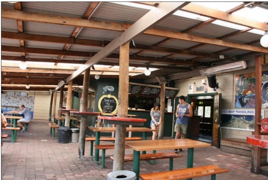
Figure 93: area beneath the large verandah addition looking to the outside bar and kitchen beyond. Weir Phillips
