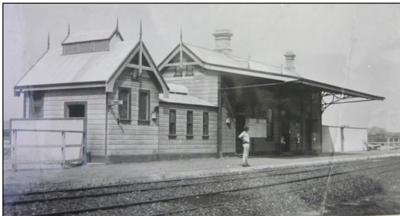
Figure 27: Undated image of Byron Bay Station. Note that the tracks are level with the platform and not in a cutting as currently shown on site. ARHSnsw
