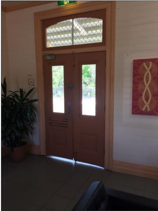
Figure 74: Timber door and joinery detail. Weir Phillips
