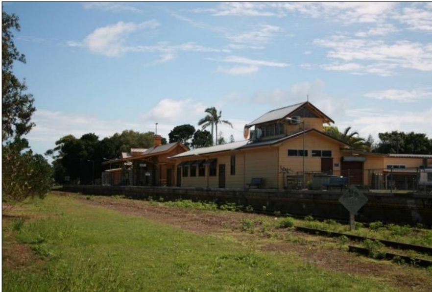
Figure 106: The western tracks have been relocated by Byron Bay Railroad Company Ltd to the north of Lawson Street. The eastern tracks remain in situ. Weir Phillips
