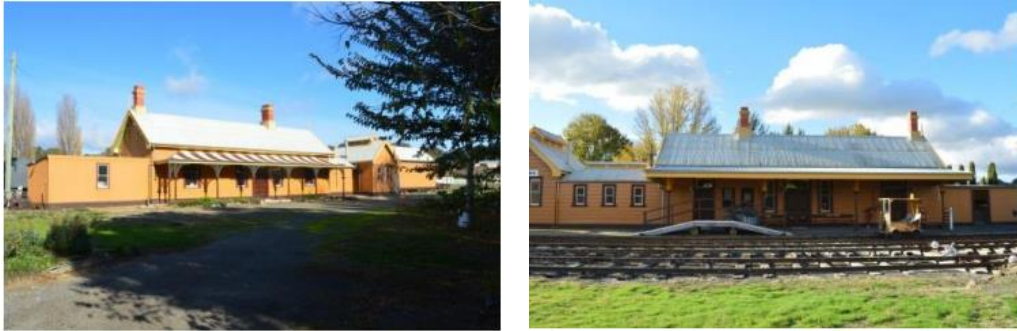
Figure 117 & 118: Yass Town Railway Station. Note the Gable ended pavillion to the left of the image. GML 2016.
