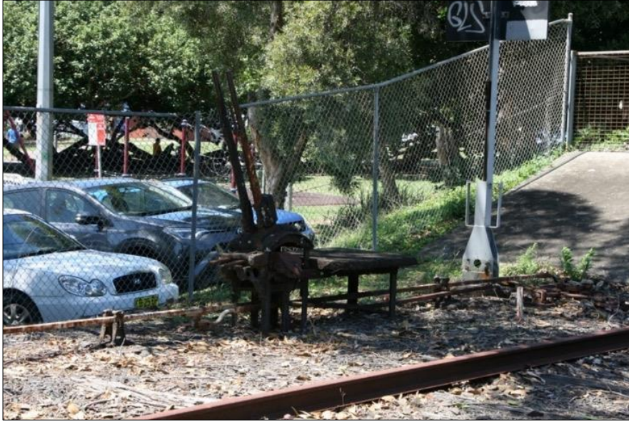
Figure 111: Eastern railway switch lever. Weir Phillips
