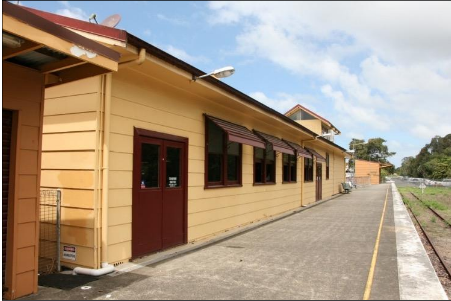
Figure 90 The railway friendly bar as viewed from the platform area. Weir Phillips
