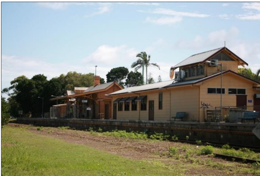
Figure 89 Western elevation of the Railway Friendly Bar and platform edge. Weir Phillips
