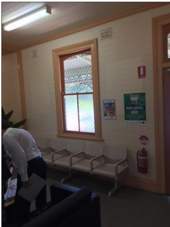
Figure 73: Original timber Sliding sash window. Weir Phillips
