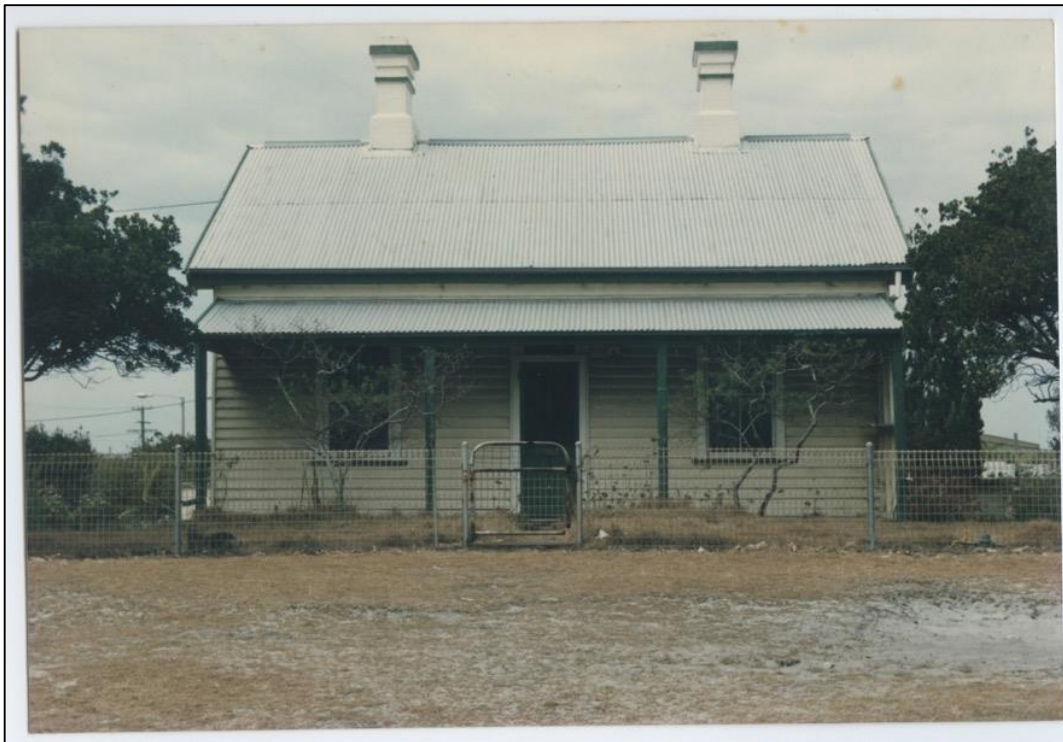
Figure 48: An undated photograph of the Station Master's House prior to its conversion to use as a Tourist Information Office. Photo courtesy of EJ Wright Collection, Byron Bay Library
