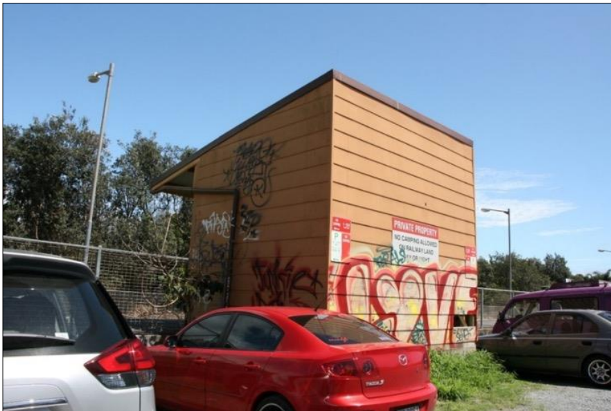
Figure 104: Eastern elevation of the Out of Shed. Weir Phillips
