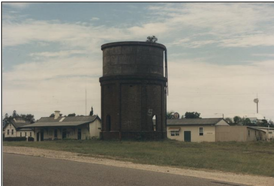
Figure 51: undated image of the water tower
