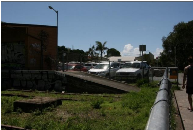
Figure 57: Pedestrian walkway to the southern boundary. Weir Phillips
