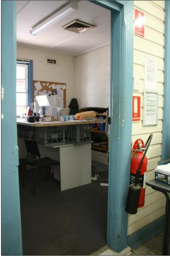
Figure 85: Office area to the rear of the building. Weir Phillips
