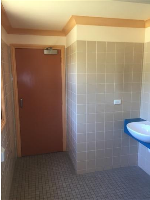
Figure 76: Modern Internal finishes noted throughout the bathrooms. Weir Phillips
