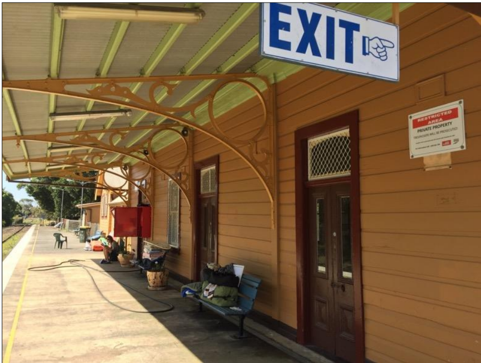
Figure 68: Former Railway Station Building detail of iron verandah supports and timber joinery details. Weir Phillips
