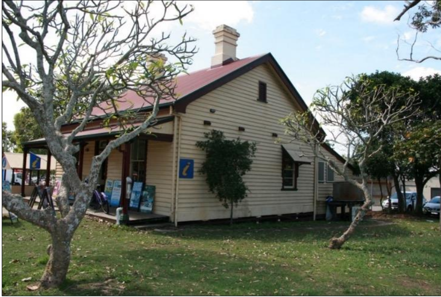
Figure 78: Western elevation of the former Station Master's House. Weir Phillips
