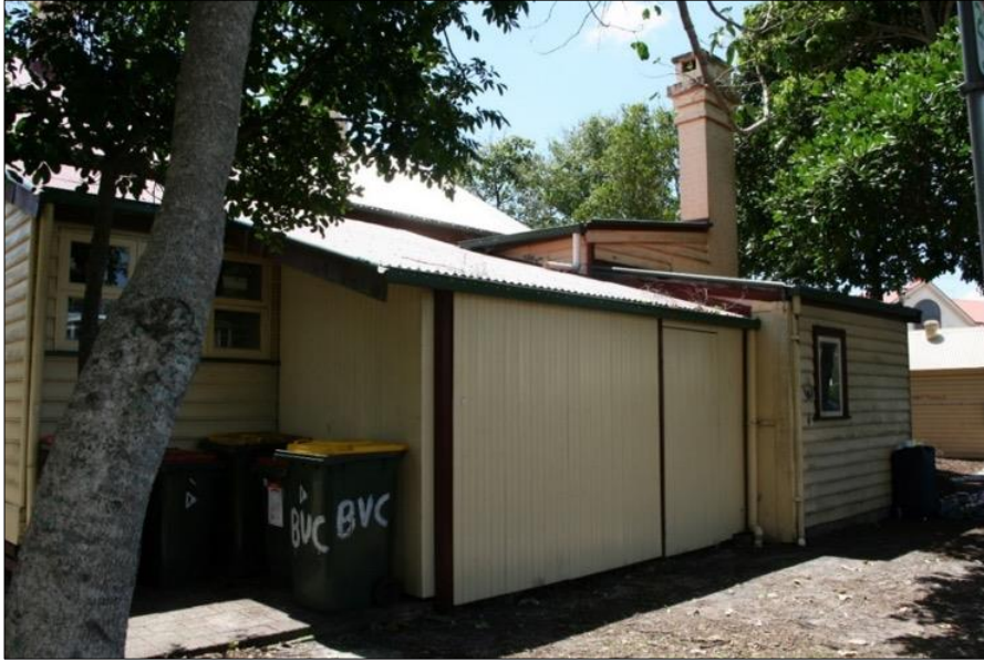
Figure 80: Rear/southern elevation with non-original lean-to extension. Weir Phillips
