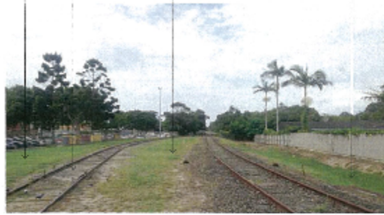
EXISTING VIEW looking south from Lawson Street end of rail corridor
