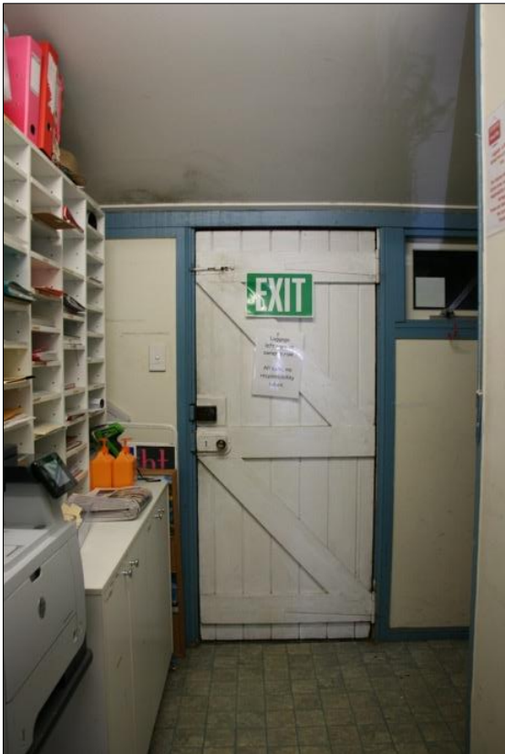
Figure 88 Rear addition. Weir Phillips
