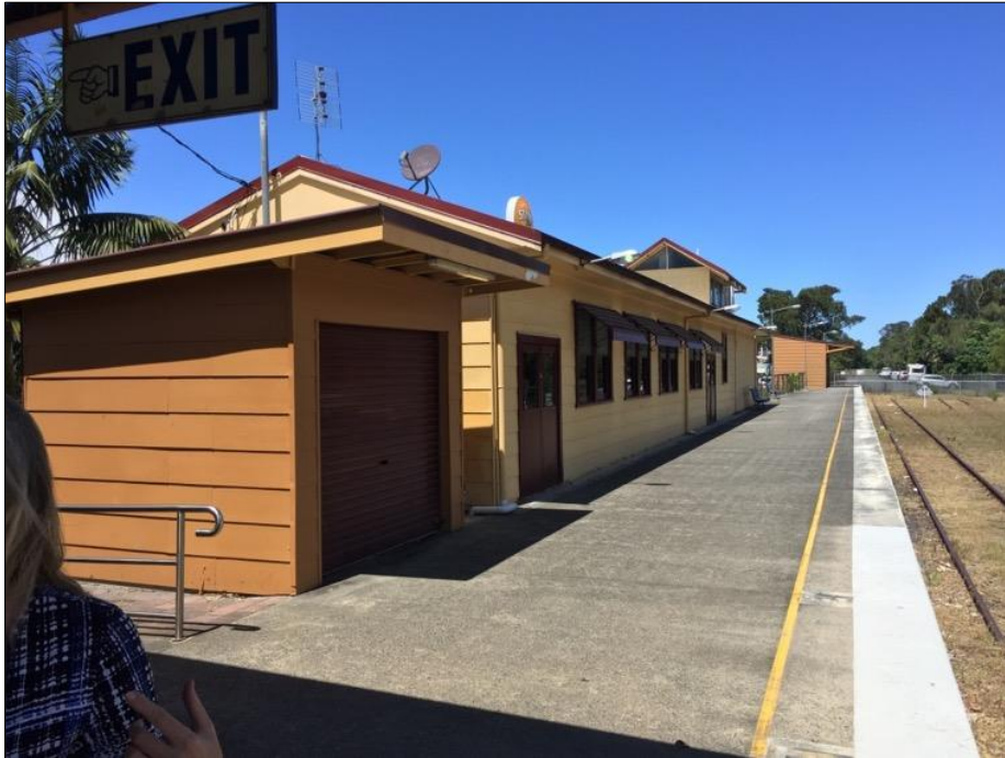
Figure 70: Storage shed and rear of Railway friendly Bar Weir Phillips
